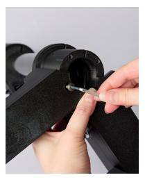
Using (1) M5x16 Bolt and the 3 mm Allen Wrench, screw the bottom of the leg to the Main Leg post. Some creaking may occur.
